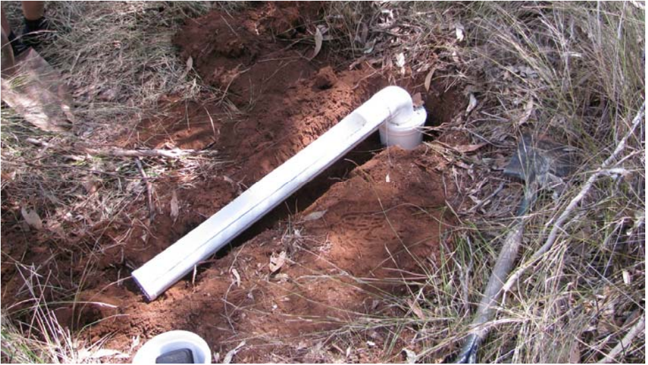
Figure 1 - A gutter trap being installed at Gurgeena Tableland. Note the dark red soil.
